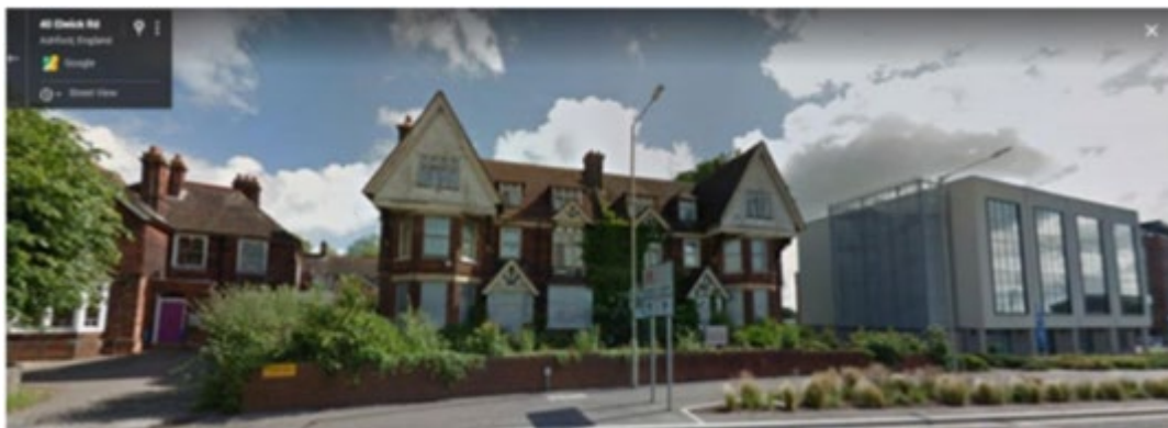
Figure 1: Frontage of Swanton House to Elwick Road
