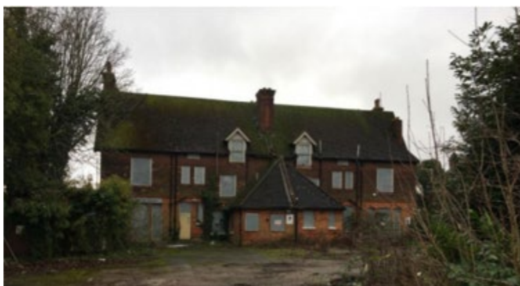
Figure 2: Rear of Swanton House
